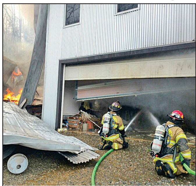
The Union County Fire Department responded last Wednesday to this structure fire off Smyrna Road, which was caused by lightning strike.
